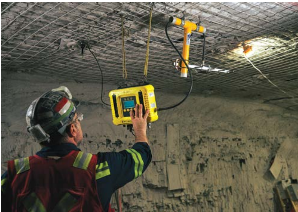
Wireless mesh communications equipment can be easily deployed (and re-deployed) to meet the changing coverage requirements in a mine. (Photo: IWT)
